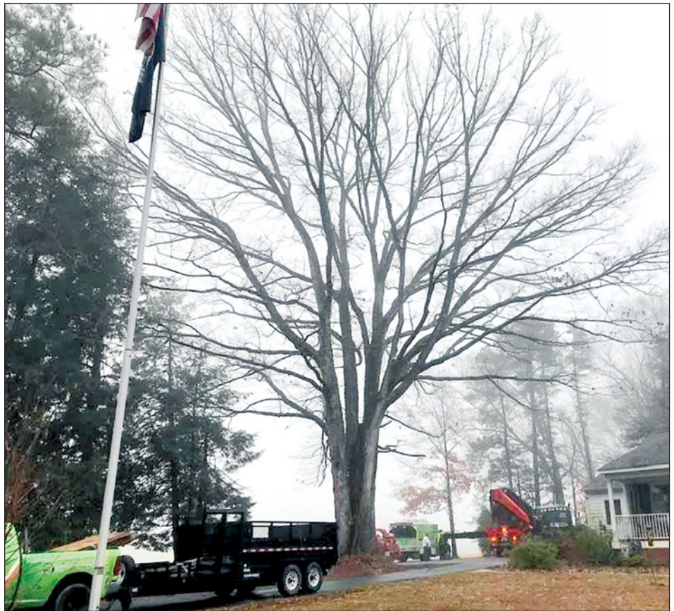
Photo 2: The job involved removing this massive white oak, Quercus alba .
