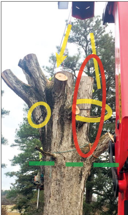
Photo 3: The yellow highlights are the lifting bridle. The green highlights show the location of the cut.
